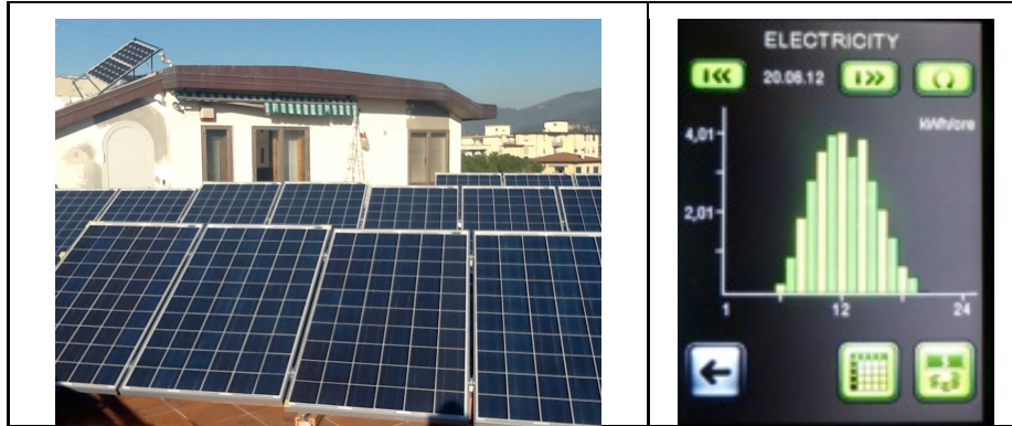
Fig. 3. Left: the terrace and roof are used for solar cell generation systems. Right: graph showing histogram of the generated energy in kWh during a sunny day on June 20, 2012.
